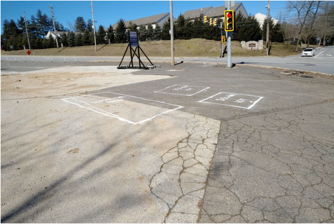
Figure 2 – Site Photograph – Detected and Field-Marked Tank Field at NE Property Corner
