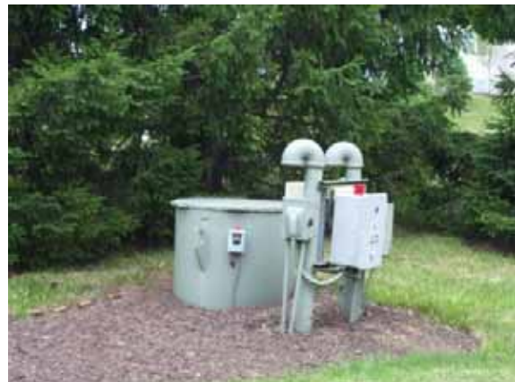
Photo #18: Sewer ejector pump
