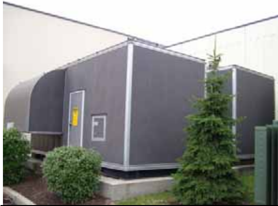
Photo #7: Natural gas fired emergency generators
