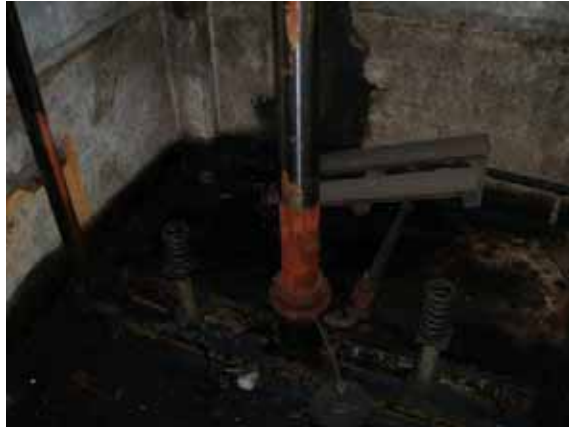
Photo #13: Severe leakage in hydraulic elevator pit
