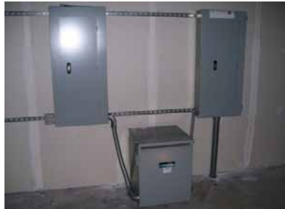
Photo #10: Dry type transformer
