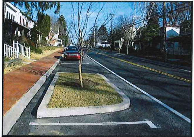
Curb bulb-outs are an effective traffic-calming device, and help to define on-street parking.
