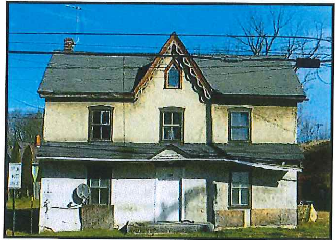
An opportunity for rehabilitation and adaptive re-use.
