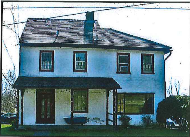
One of the several intact buildings in Guthriesville that could be adaptively re-used.
