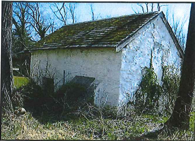
Historic accessory building (spring house) provides an opportunity for adaptive re-use.
