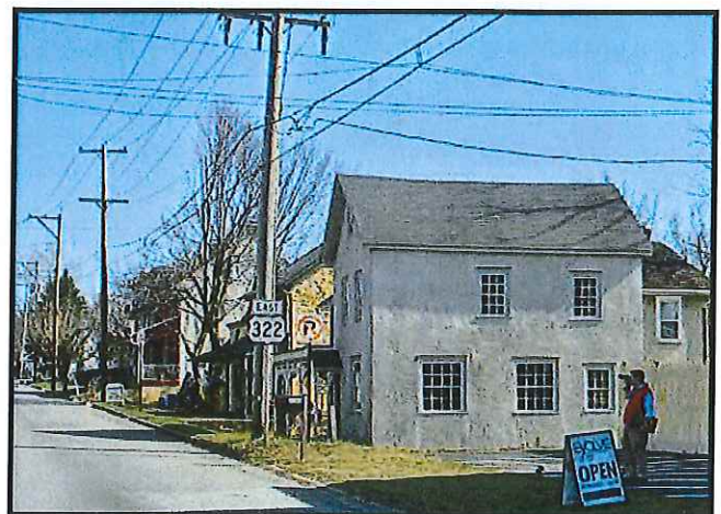
Existing buildings in alignment along Route 322.
