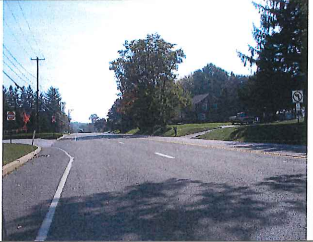
Route 322 looking south
