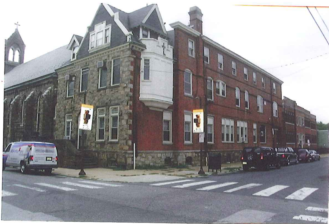
CONVENT BUILDING FRONT AND WESTERLY ELEVATION
