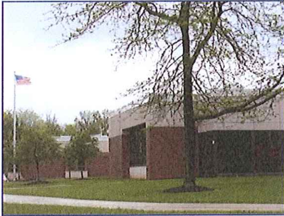
Boyertown Area Jr. High East Center
