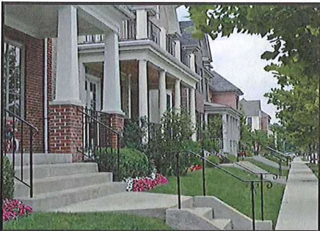
New buildings in alignment along the streetscape.
