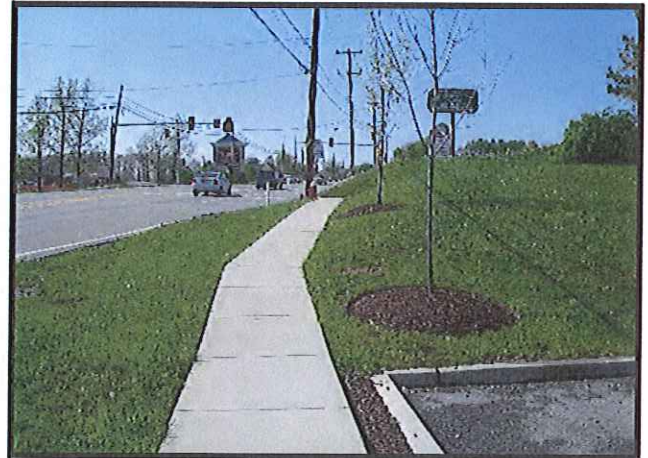
A well-maintained sidewalk along the base of a slope/berm as part of a network of pedestrian connections.
