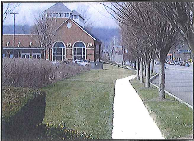
Street Trees with upright form along the streetscape (with retail building located close to the sidewalk).
