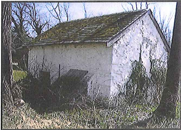
Historic accessory building (spring house) provides an opportunity for adaptive re-use.
