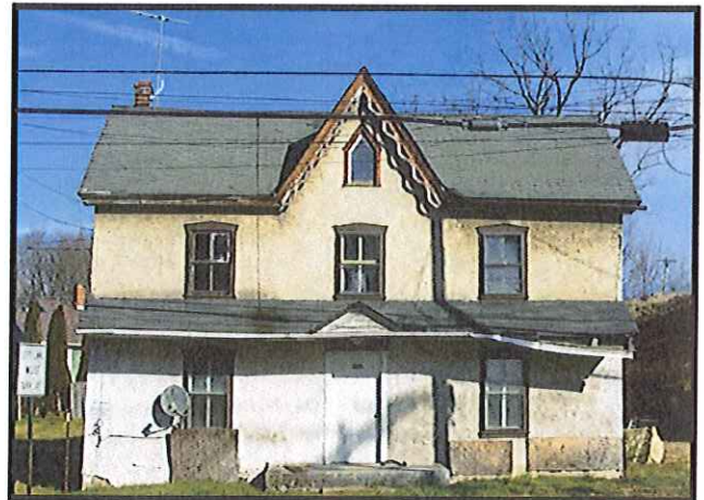
An opportunity for rehabilitation and adaptive re-use.
