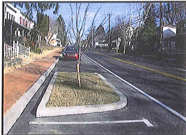
Curb bulb-outs are an effective traffic-calming device, and help to define on-street parking.
