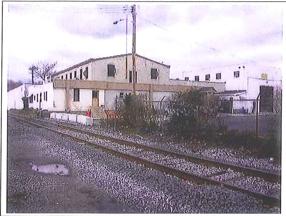
VIEW TOWARDS JEFFREY ST BUILDING ELEVATIONS
