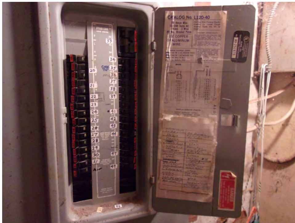
Photograph 11 - Picture of a circuit panel in the farmhouse basement.
