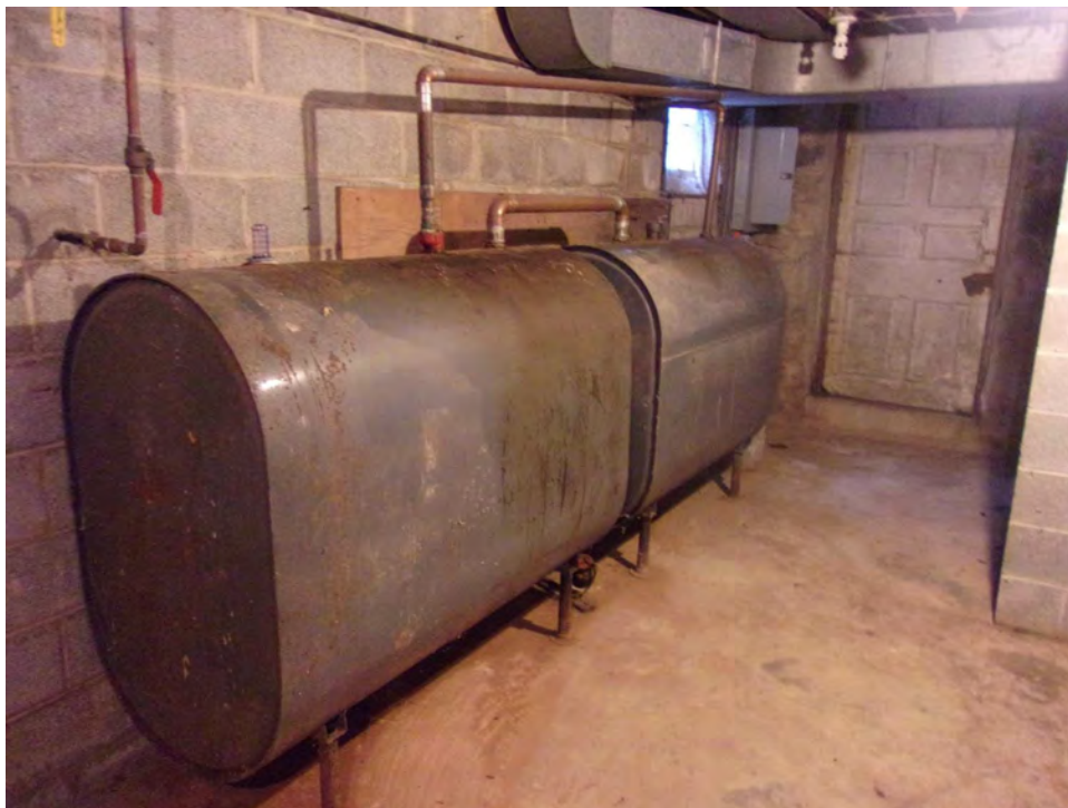
Photograph 9 – View of two 275-gallon aboveground heating oil tanks in the farmhouse basement.
