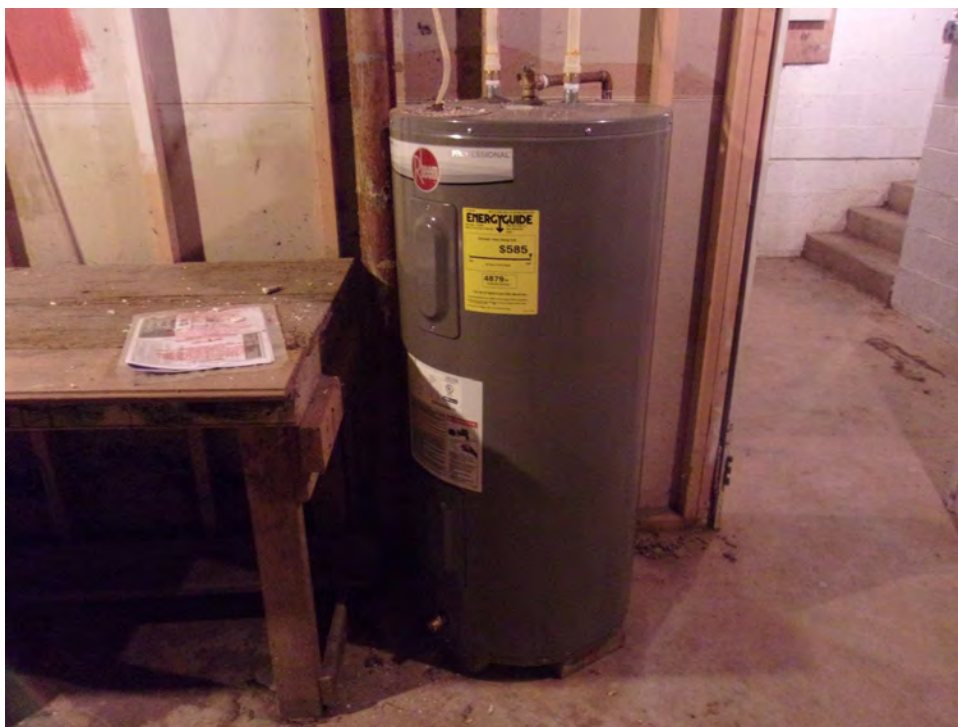
Photograph 10 – Photo of a water heater in the basement.
