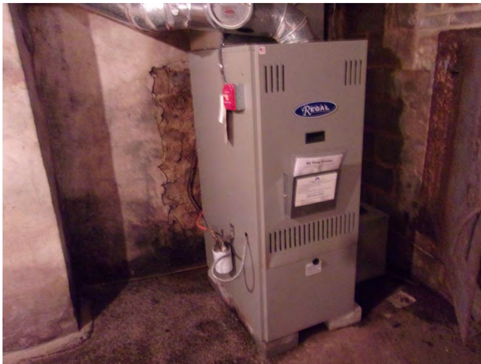
Photograph 8 – Picture of an oil fired furnace in the farmhouse basement.
