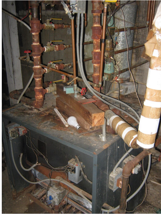
Natural gas fired furnace for converted barn dwelling
