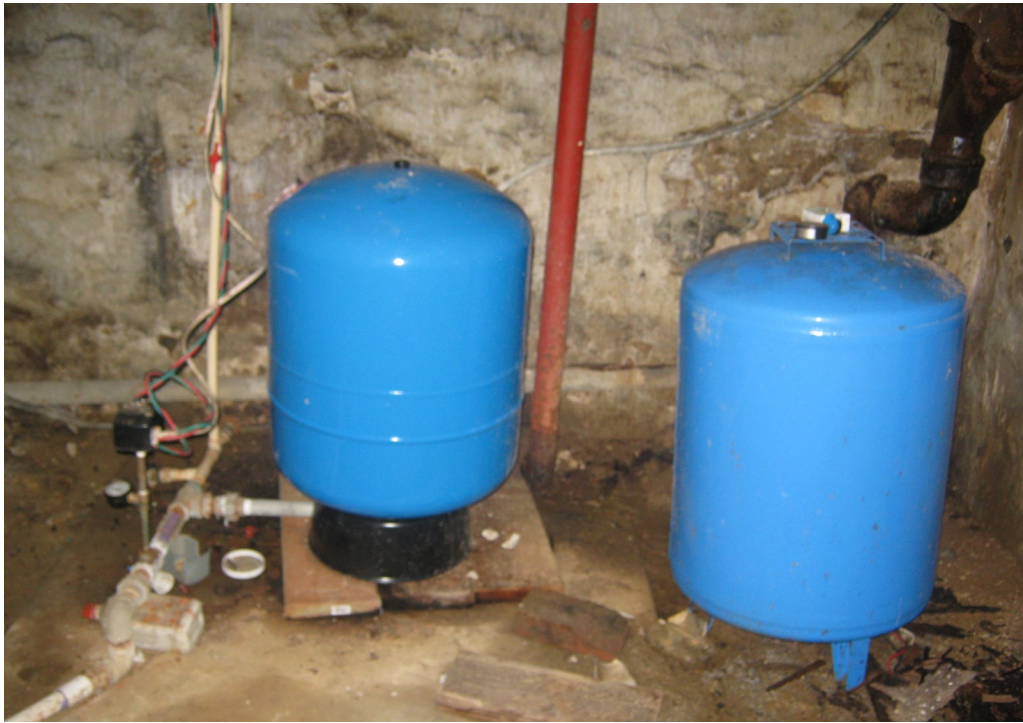
Well pressure tank in basement of 3 story dwelling
