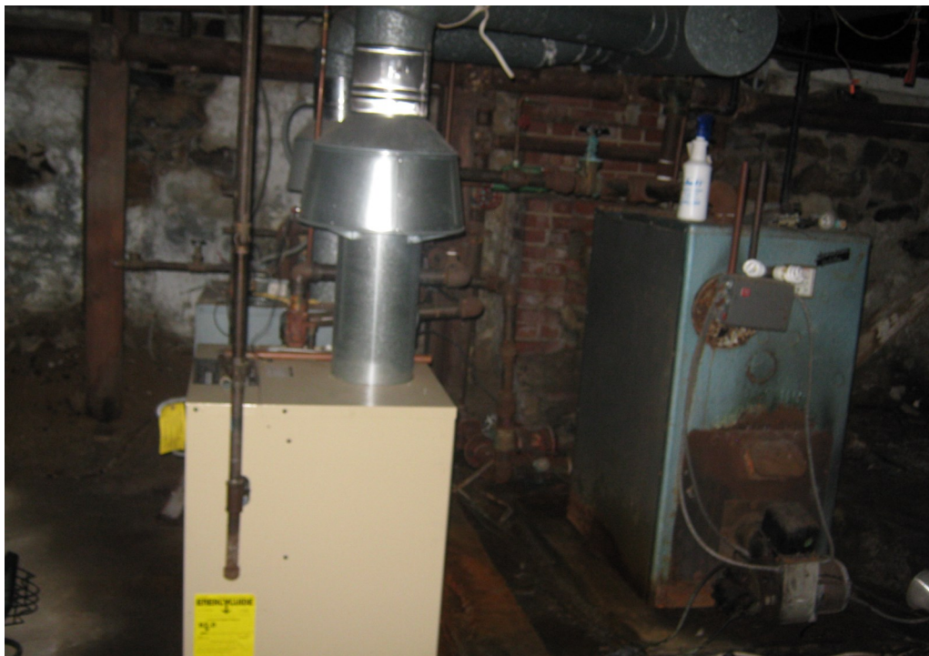
Natural gas fired furnace in basement of 3 story dwelling
