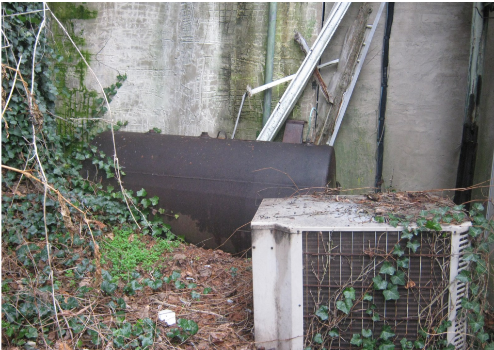
Empty heating oil tank for former heating oil furnace at converted barn dwelling
